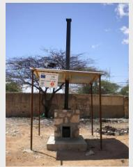
Fig. B.2 – New De Montfort incinerator built at General Group Hospital
